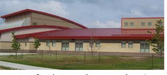
In most retrofit projects, standing seam roofs can be installed right over existing built-up roofs, eliminating costly and time consuming removal. The metal panels are attached to steel framing to provide a sloping surface to effectively shed rain and snow. Standing seam panels are available in a wide range of standard pre-finished colours, in addition to galvalume. The WS-2401-20" Standing Seam Roof System (SSR) includes a 20 year warranty.
